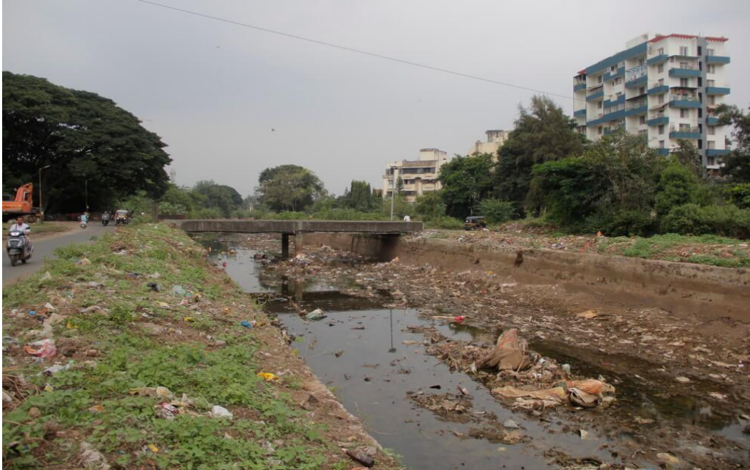
The Mula-Mutha has been steadily reduced to a large sewer, randomly concrete-fenced, prone to flooding and clogging with the city's waste. Photo: Ishan Sadwelka
