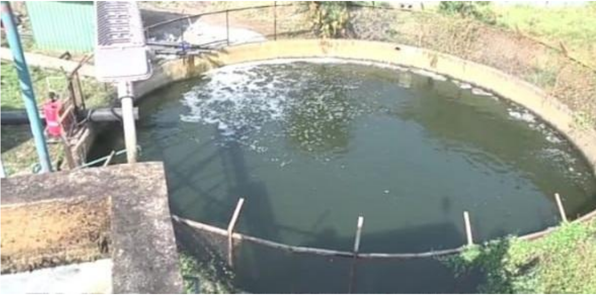
Circular Untreated River Water Inlet Tank
